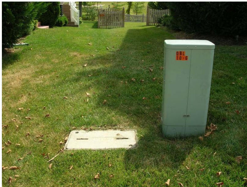
Figure 5: Telephone Pedestal with CATV and Fiber Optic Vault for HSD
