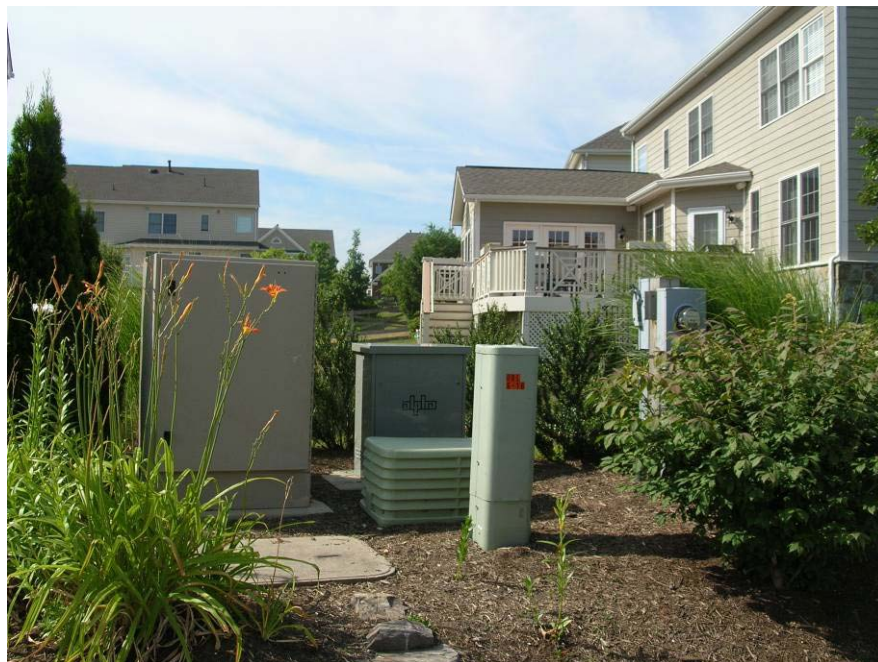
Figure 8: Location Illustrating AON Equipment, Power Supply, Node, and Telephony
