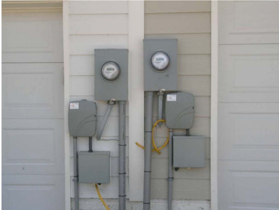
Figure 9: Location Illustrating the PON Equipment at a Subscriber Townhouse
